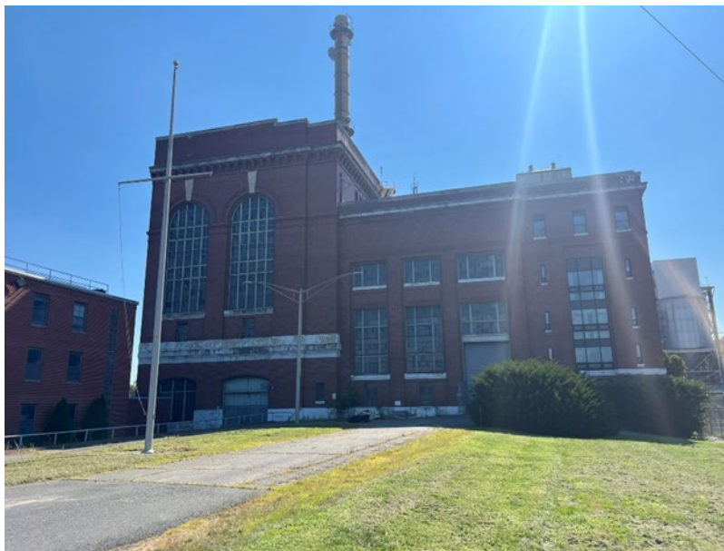
Figure 3-17. View of the north elevation of the building today, with the historic portion seen on the right-hand side Source: Weston & Sampson site visit, 2024
