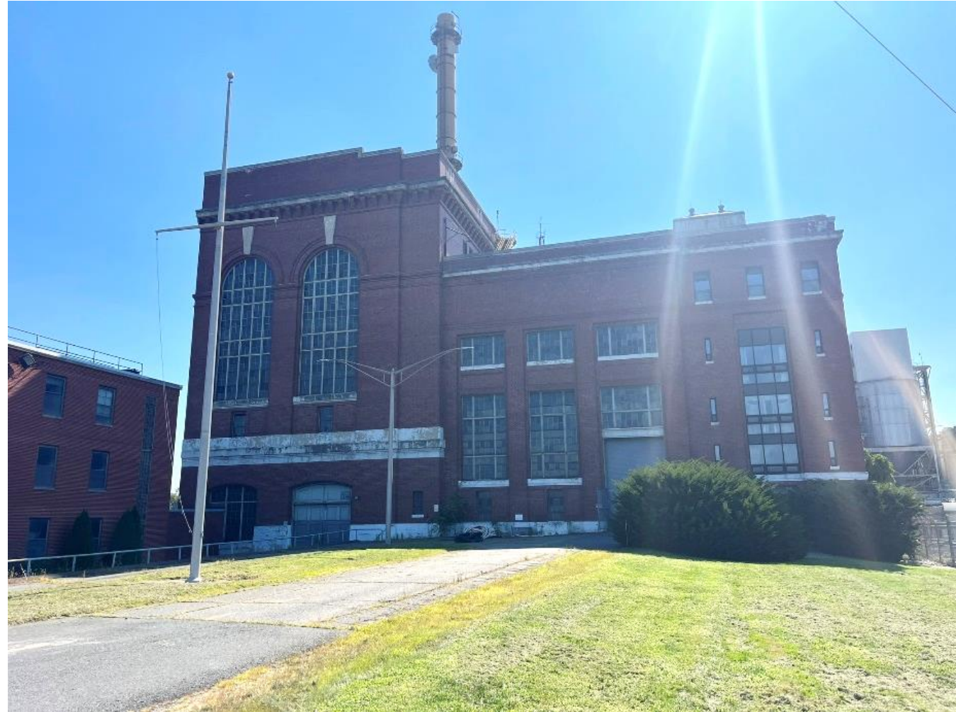
View of the north elevation of the building today, with the historic portion seen on the right hand side Source: Weston & Sampson site visit, 2024
