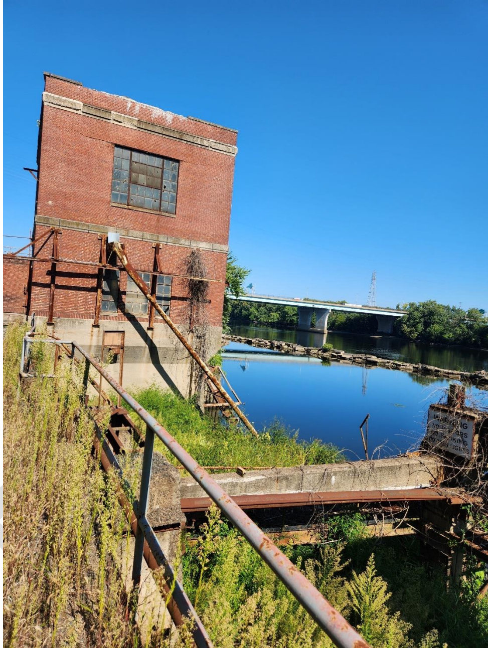
Figure 4-2. Screen houses on the Connecticut River Source: Weston & Sampson site visit, 2024
