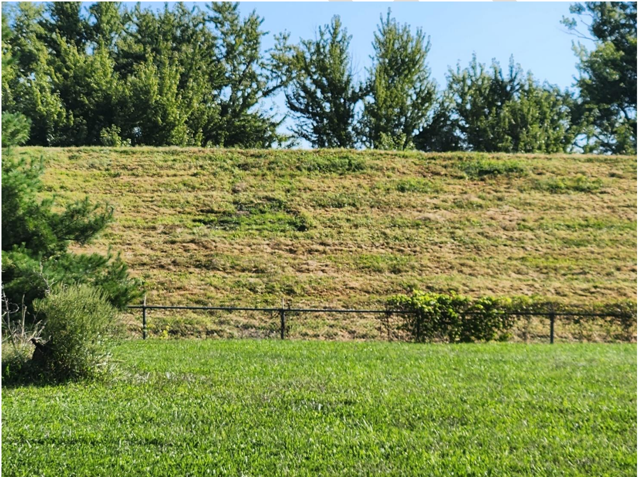
Figure 3-3. Earthen dike component of levee Source: Weston & Sampson site visit, 2024
