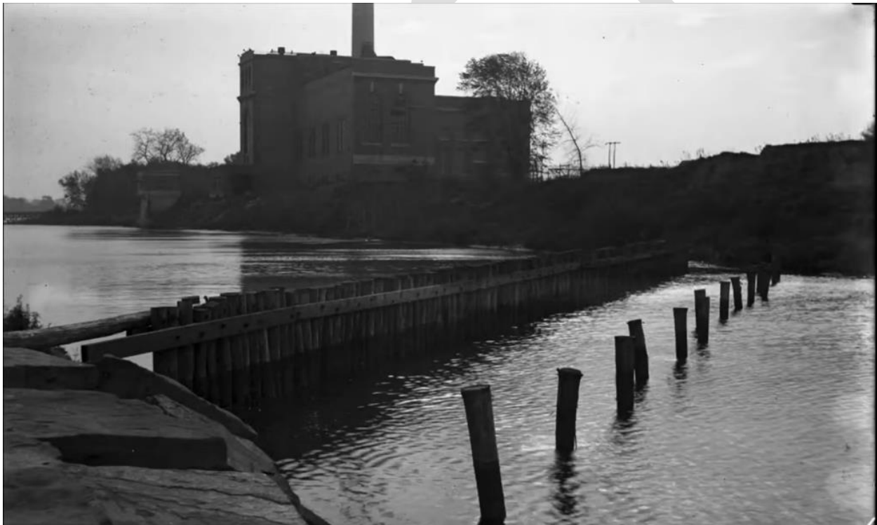
Figure 4-10. View of the South Meadow Power Plant from the Connecticut River in 1922 Source: Hartford History Center, Hartford Public Library
