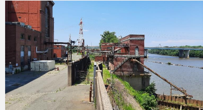
Flood Control Dike on Site.
