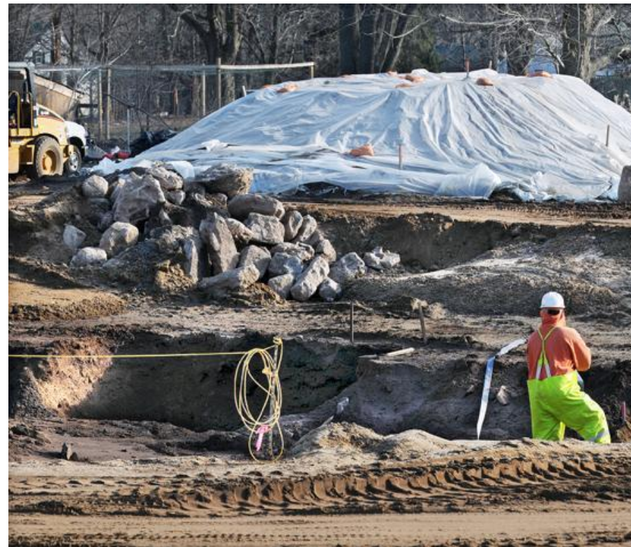
Site cleanup at the Durham Meadows Superfund Site. Photo by W&S
